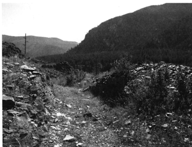
Figure 4. Mullan detailed a 150-man crew to carve the Point of Rocks and Big Side Cut sections of the wagon road from the mountainside above the Clark Fork River. Although Mullan claimed in 1863 that all the cuts were fifteen to twenty feet in width, some, like this one, were much narrower. This cut is seven feet wide. Photo by Jon Axline.
