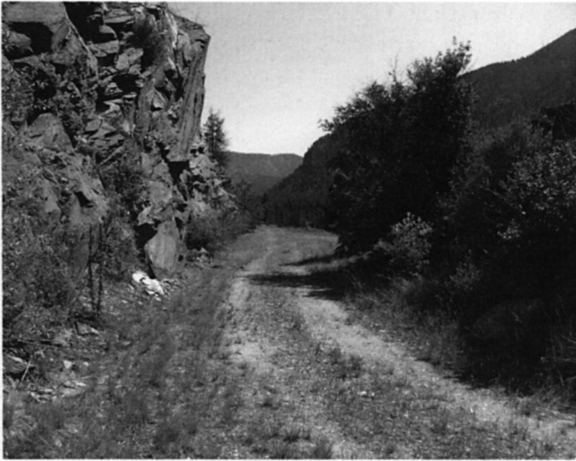
Figure 9. The Milwaukee Road was forced to remove an enormous amount of rock to maintain its two percent grade as it approached the summit of the Bitterroot Mountains to the west. Photo by Jon Axline.
